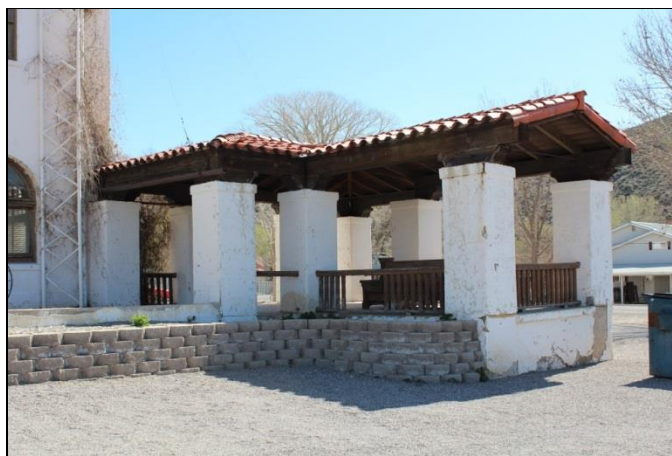
Figure 38. A general view of the pergola, view facing north.
