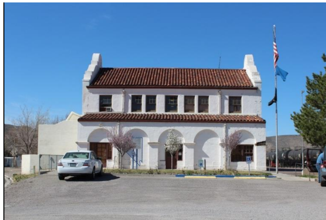
Figure 2. Northeast side of Caliente Depot, 2015.
