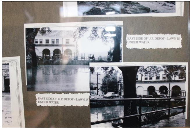
Figure 8. Undated image (ca. 1930s) of Caliente Railroad Depot before full enclosure of the northeast arcade. Note the light paint color of windows. Courtesy City of Caliente Boxcar Museum.
