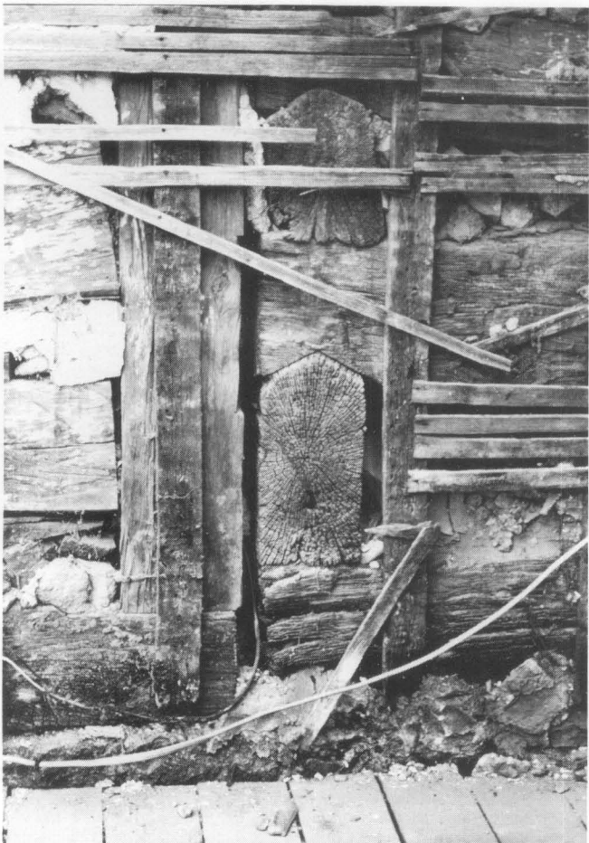
Fig. 8. Removal of deteriorated stucco in preparation for stucco repair on this late-18th century log house in Middleway, West Virginia, reveals that the stucco was applied to hand-riven wood lath nailed over vertical wood strips attached to the logs. Photo: Anne Grimmer.
