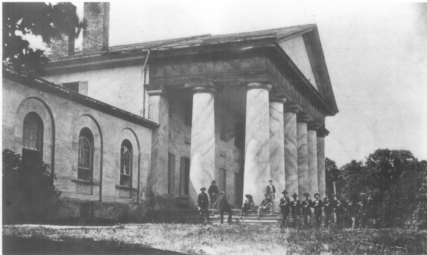
Fig. 6. Arlington House, Arlington, Virginia, was built between 1802–1818 of brick covered with stucco. It was designed by George Hadfield for George Washington Parke Custis, grandson of Martha Washington, and was later the home of Robert E. Lee. This photograph taken on June 28, 1864, by Captain Andrew J. Russell, a U.S. Signal Corps photographer, shows the stucco after it had been marbled during the 1850's. Yellow ochre and burnt umber pigments were combined to imitate Sienna marble, and the stucco, with the exception of the roughcast foundation, was scored to heighten the illusion of stone. Photo: National Archives, Arlington House Collection, National Park Service.
