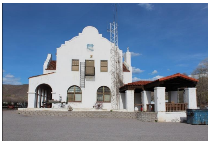
Figure 4. Southwest side of Caliente Depot, 2015.
